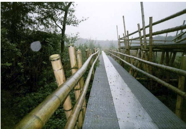
Fig. 7. Bamboo bridge in the Amsterdam Woods [photo: Pablo van der Lugt].
